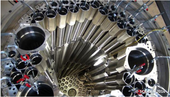
Fig. 4. The BR2 reactor with a Be moderator tubes 2
